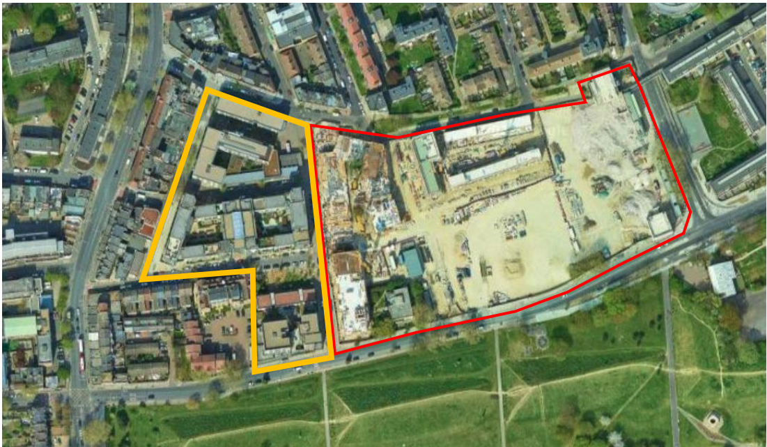
Figure 1.8: Aerial photograph showing the location of Site 1A (orange) adjacent to the FDS (red)
